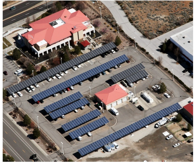
Sparks Police Department Photovoltaic Project
